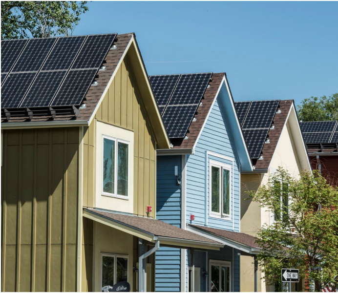
Solar panels atop homes in Boulder, CO
